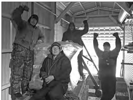
The hard-working crew of Victor Keene, Will Peterson, Edward Twitchell and Harold Pavilla celebrate moving the engine into place to await installation. A big thank you to all involved!
