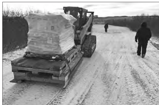
A Bobcat pulled the engine to the power plant over an icy road.
