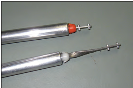
Top, tilt-in, double-hung window sashes may need spring adjustment to stay up.
