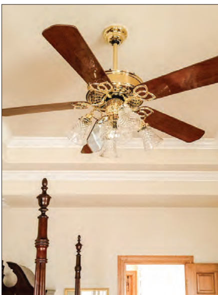
In the winter, reverse the spin of your ceiling fan and set it on the slowest speed to help send warm air into the room.
