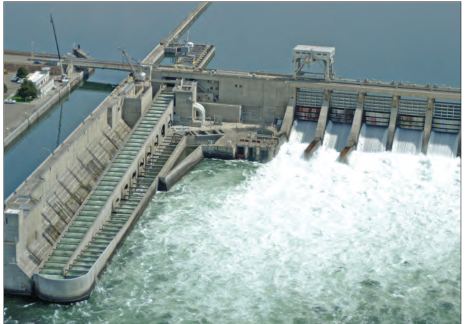
McNary Dam on the Columbia River is one of eight Snake and Columbia river dams ordered to increase the amount of water spilled rather than used to produce electricity. The U.S. Court of Appeals for the Ninth Circuit ordered more water to be spilled over the region's dams to help migrating salmon.
