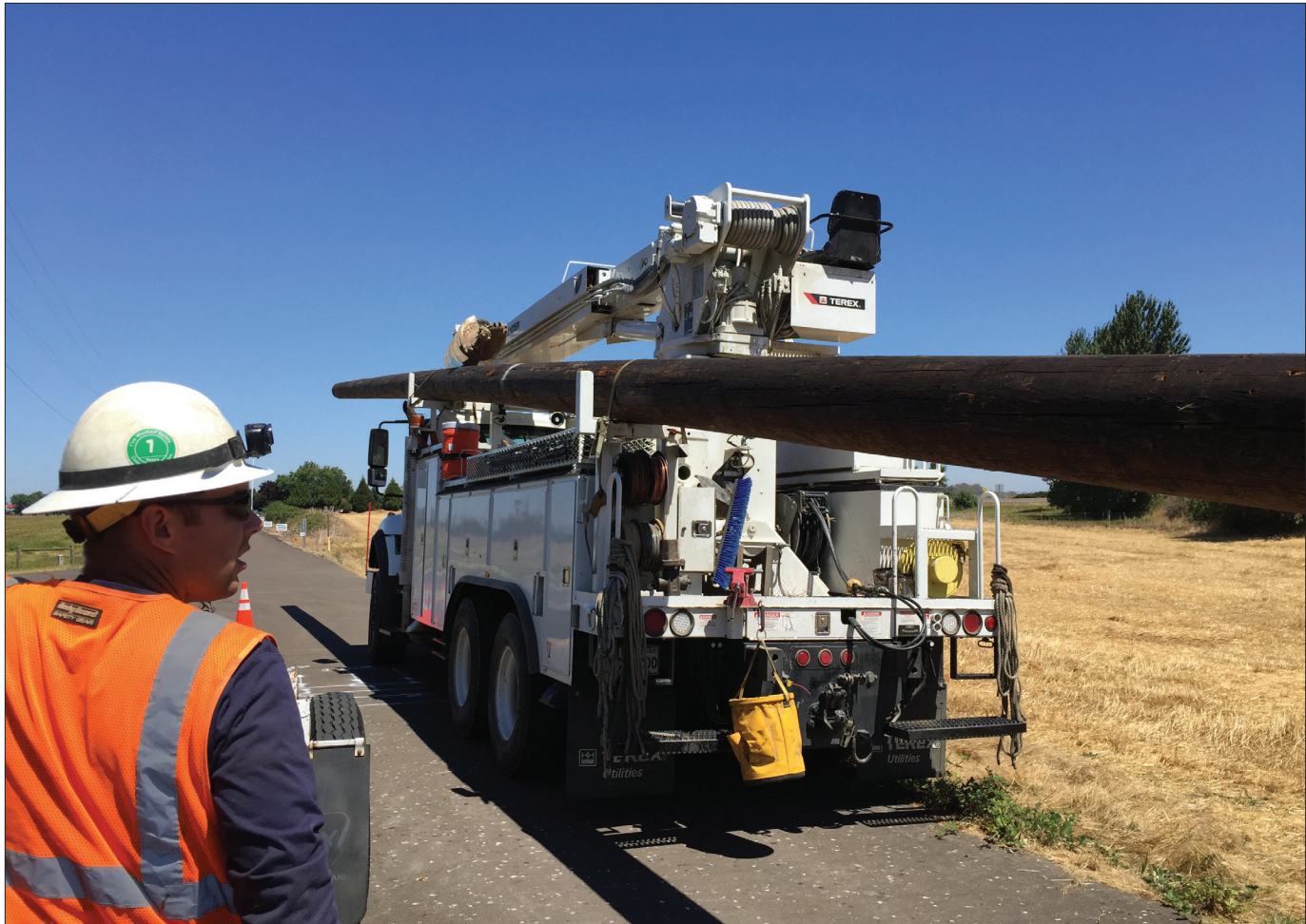
Foreman Brad Jarmain oversees work for a pole replacement.
