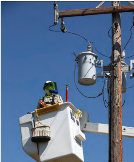
Above, a serviceman wears a face shield, fire-resistant shirt and protective gloves while checking a transformer. Right, lineworkers prepare to replace insulators on a 69-kilovolt line.
