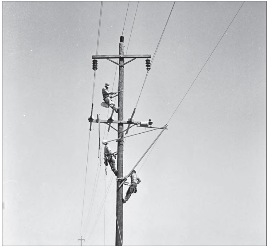
Above, a serviceman wears a face shield, fire-resistant shirt and protective gloves while checking a transformer. Right, lineworkers prepare to replace insulators on a 69-kilovolt line.
