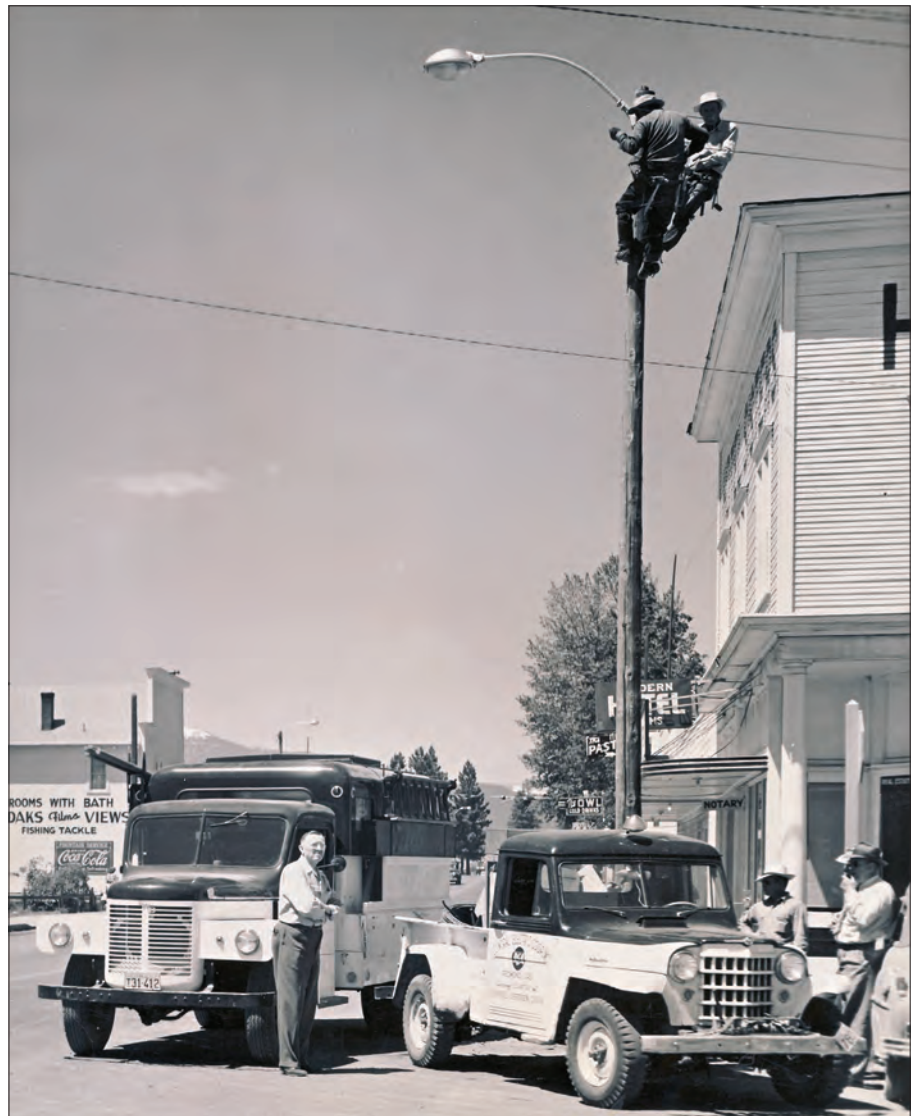
Linemen work on a street light in Sisters in 1949.
