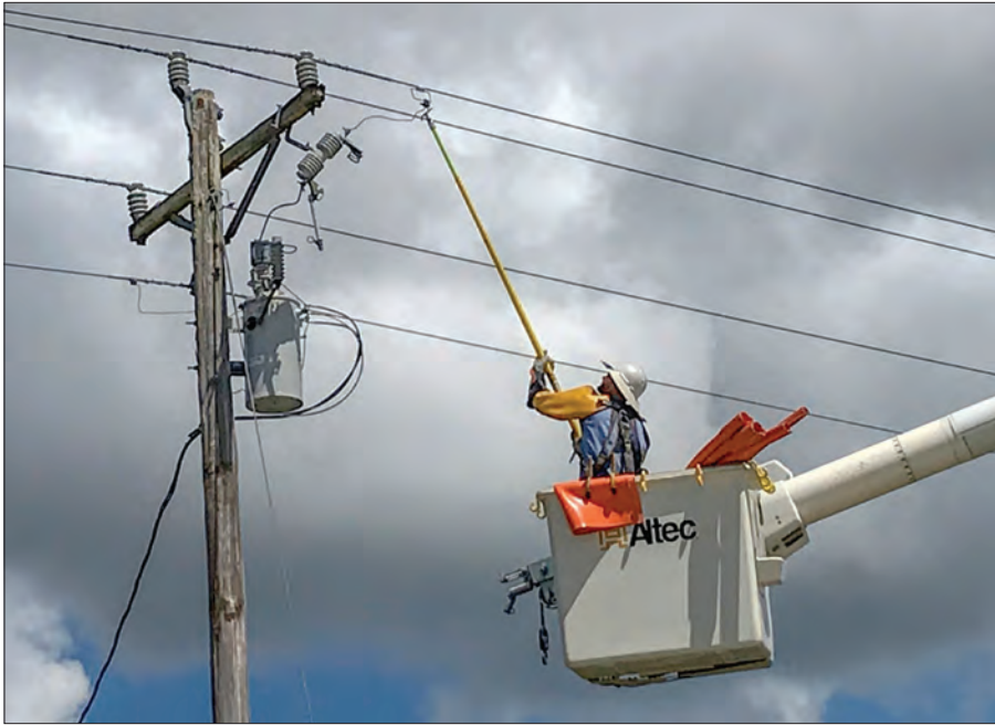
Glades Electric Cooperative Journeyman Lineman Greg Culbertson uses a hot stick to change out electrical equipment on a distribution line. The crew was working along Grand Concourse in Highlands County.
