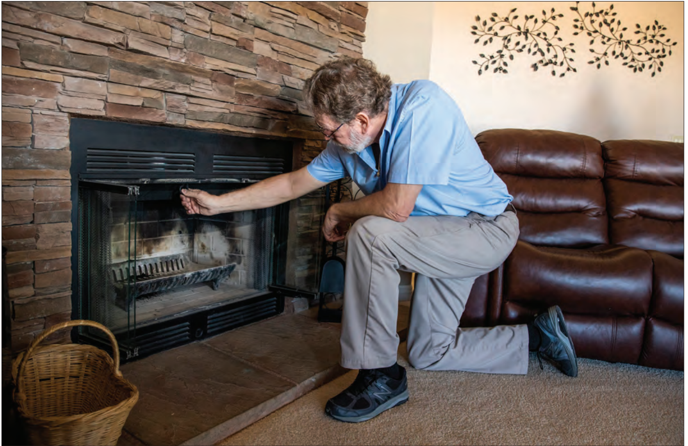
Make certain the fireplace damper is closed when not in use.
