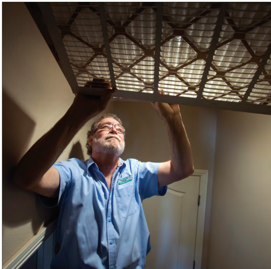
Replacing air filters as VEA member Carl Hereford is doing here can increase airflow, improve comfort in the home and reduce costs.
