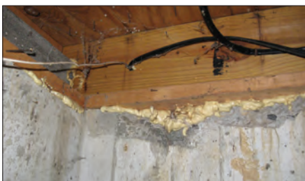
Use expanding insulating foam to seal wiring holes and gaps where the sill plate rests on the foundation.
