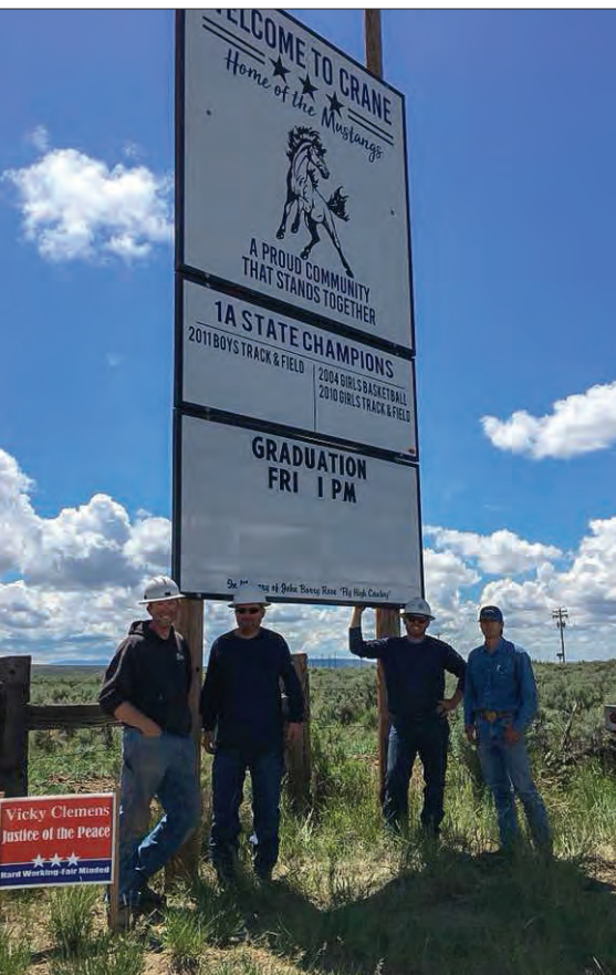
Linemen from Harney Electric based in Hines, Oregon, helped install a new sign for Crane schools.
