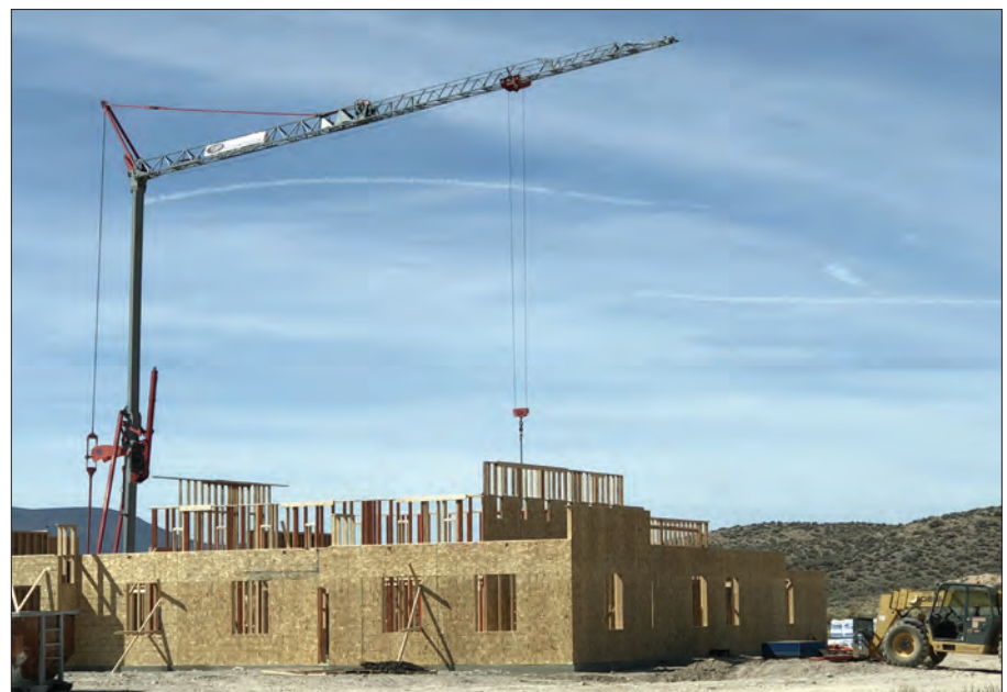
The headquarters building under construction in September.
