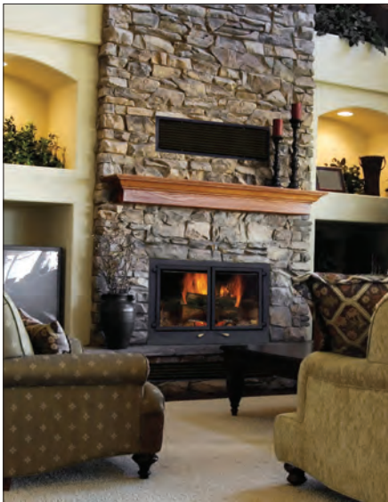
Decorative airtight doors on this heat-circulating fireplace improve efficiency and reduce air loss.
