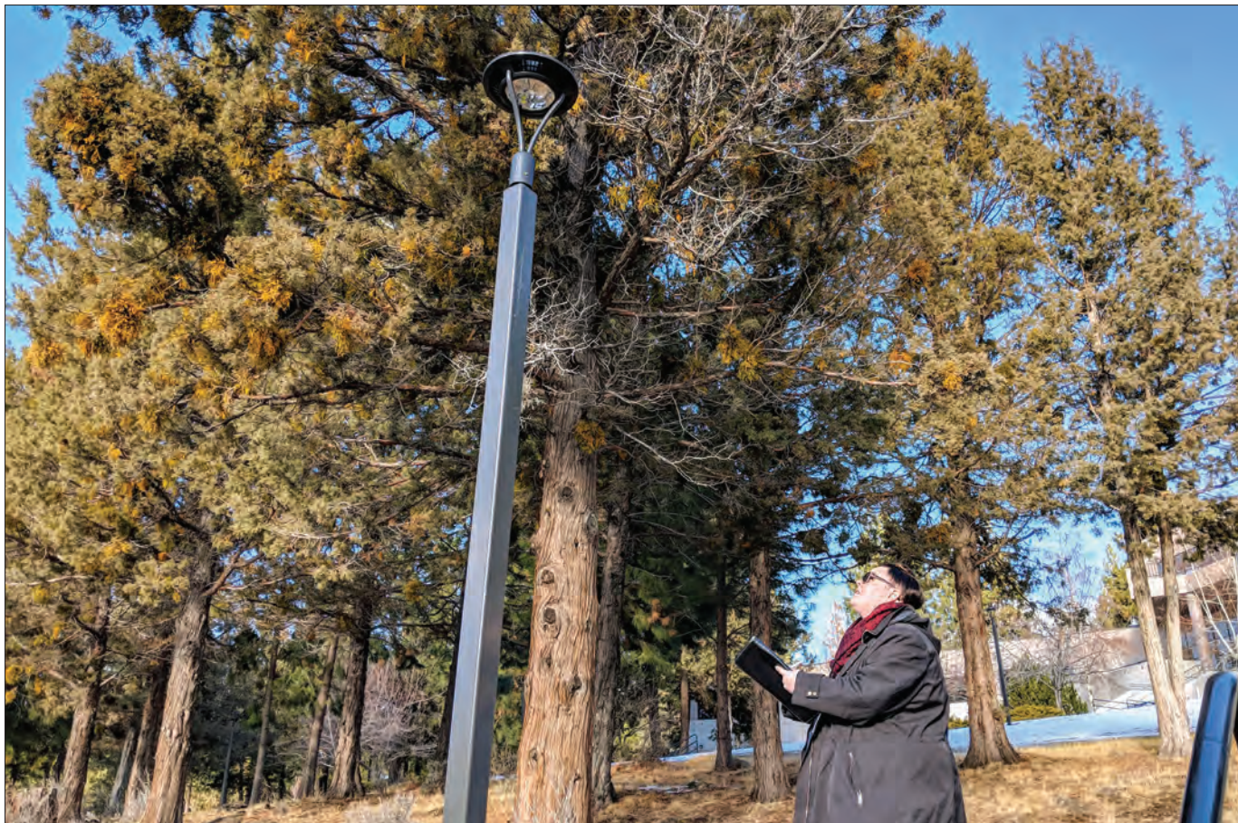
Evergreen Consulting Group/CEC Lighting Specialist Kandis Bray inspects a recent lighting installation in Central Oregon.
