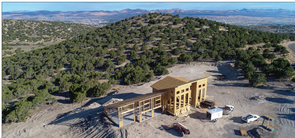
A construction site in Northern Nevada photographed by Rick and Talon 1.
