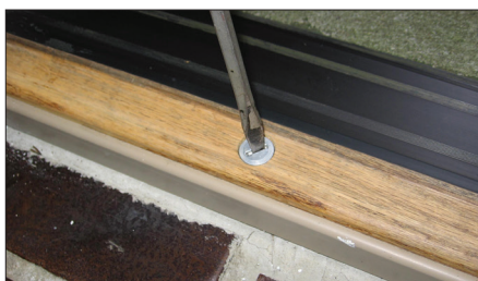
The threshold under the door can be raised or lowered with a screwdriver so the door bottom weatherstripping seals tightly.
