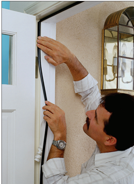
Replaceable vinyl weatherstripping seals well on the hinge side of the door because it gets compressed with little rubbing and wear.
