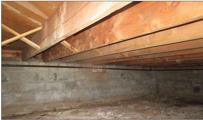
Above, the floor of the Kuehns' home had no insulation when they moved in. Right, Mike Stewart added a heat pump water heater to his home, reducing his water heating costs significantly.
