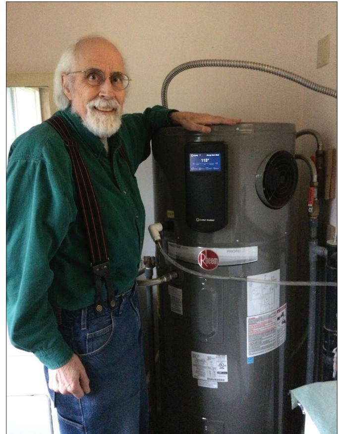
Above, the floor of the Kuehns' home had no insulation when they moved in. Right, Mike Stewart added a heat pump water heater to his home, reducing his water heating costs significantly.
