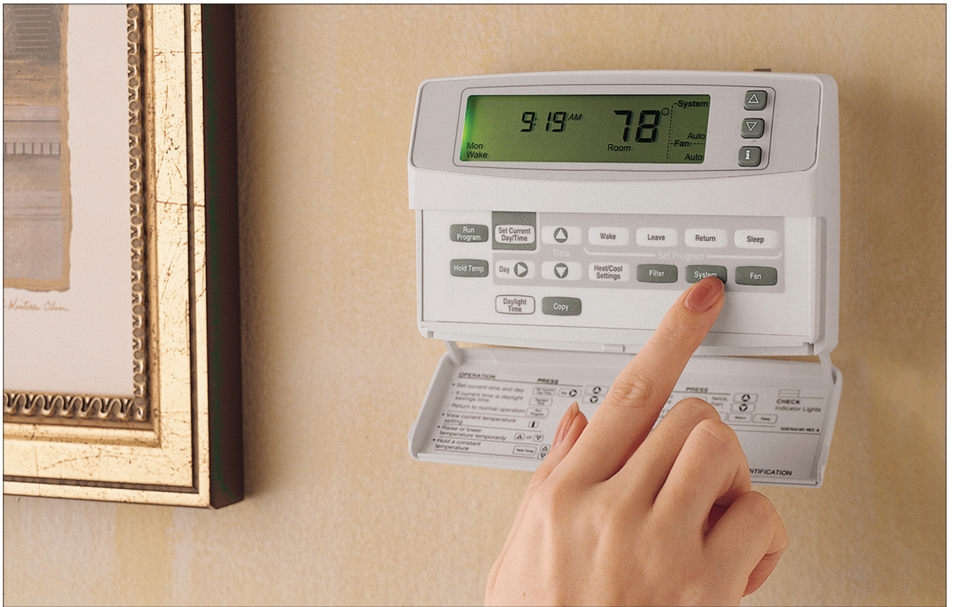
Programmable thermostats help homeowners control when their heating and cooling systems run, but they cannot control how hard the HVAC system has to work.
