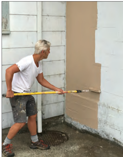
Eric painting the outside of the building.
