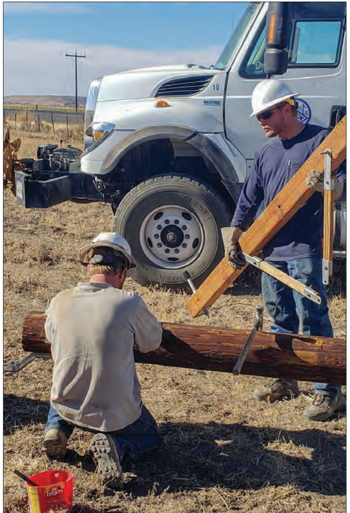
Clockwise from top left, HEC crews install a new transmission switch. Wyatt Shelley replaces a transmission arm. Mitchell Ebar and Jeff Pyburn frame a pole for a new irrigation service. Jason Rankin works on a new irrigation service.
