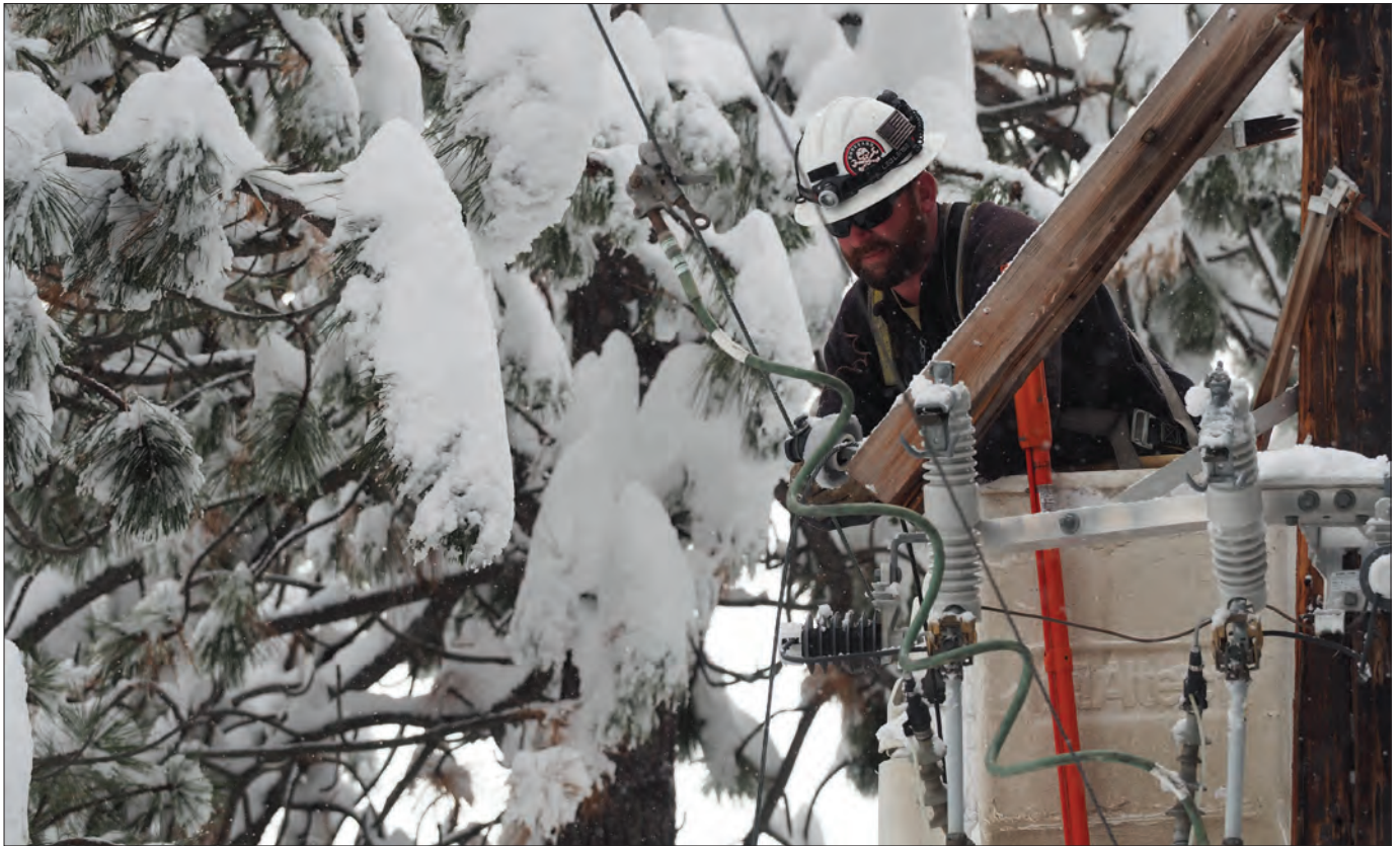
Serviceman Eric Youngstrom fixes a broken crossarm in Sisters.
