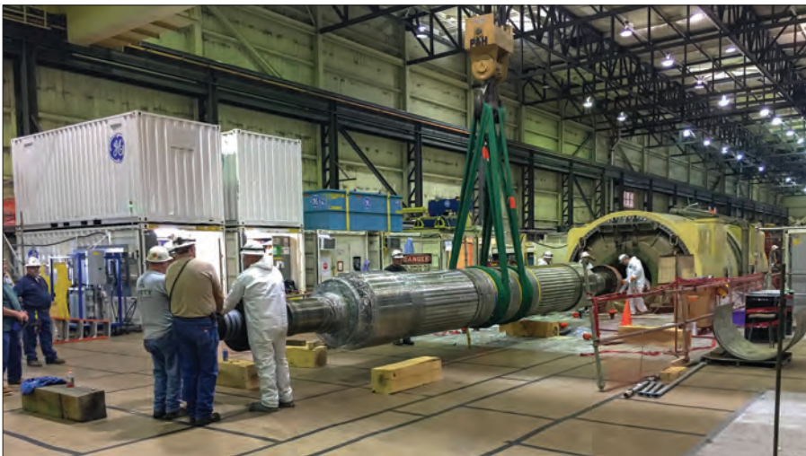
When it comes to electric reliability, the biggest challenge is maintaining and updating the massive machinery that makes up the nation’s electric grid.
