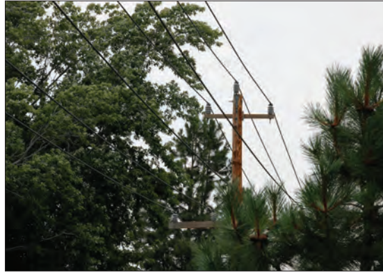
Left, if you have trees growing into power lines report it to CEC right away.
