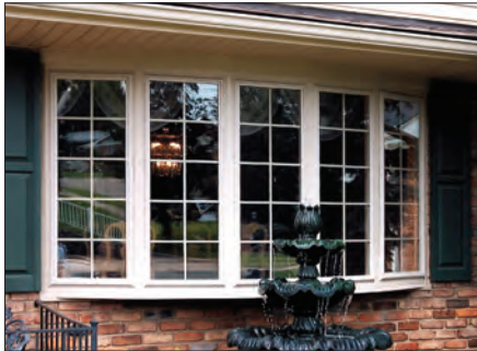
This five-section bow window with a vinyl frame has casement windows on either end for maximum natural ventilation.
