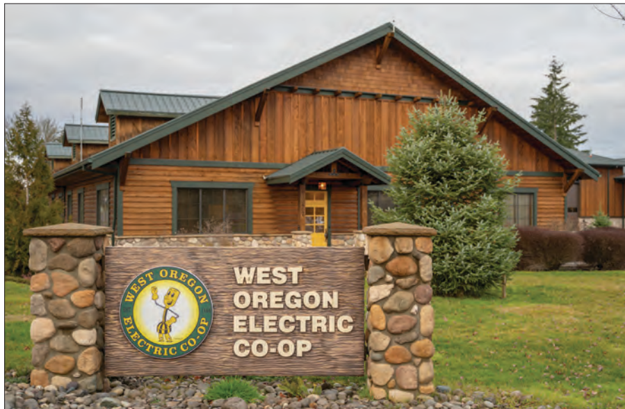
WOEC's current headquarters were built on higher ground in 2011 to avoid future damage from floods.
