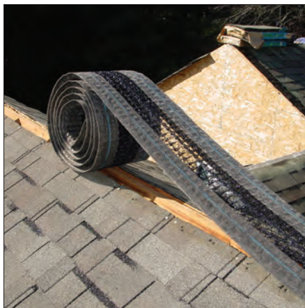
Roll out the ridge vent, smooth it down and cut it to length.
