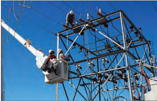
CEC linemen make system upgrades at the Hampton Substation.
