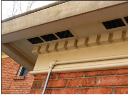
Install half of the required vent area in soffit vents. These are 4-by-16-inch vents.
