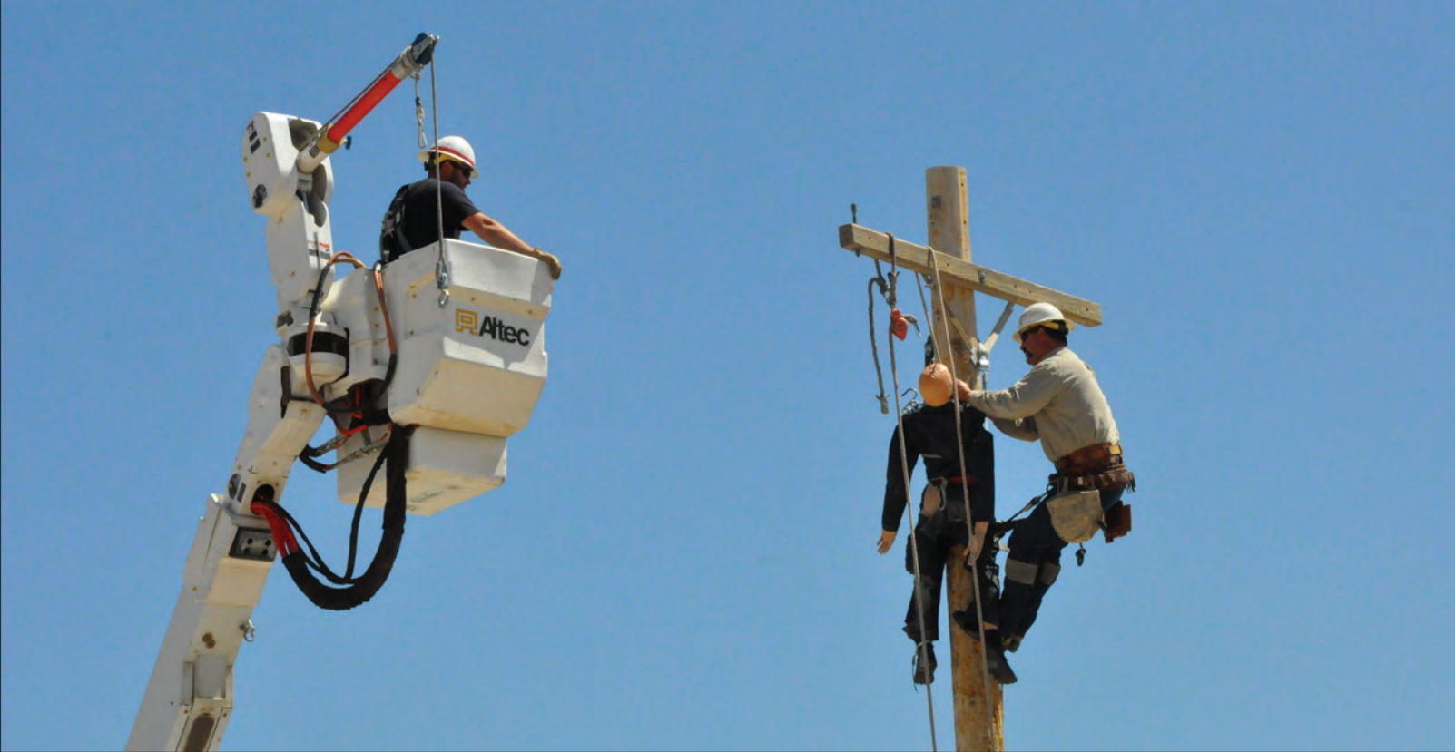
Mt. Wheeler Power Linemen Bill Baumann, right, and Jason McNutt conduct a pole-top-rescue training exercise. Photo by Christina Sawyer
