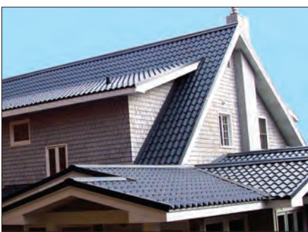
This simulated tile roof is made from painted steel. Many stock colors are available.
