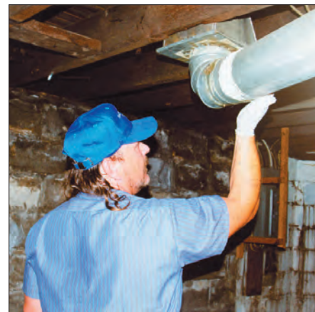
Check ducts. Seal any openings with mastic tape.
