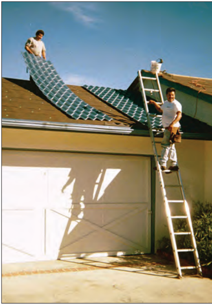
Each large metal roofing panel covers a large area of the roof for simpler installation
