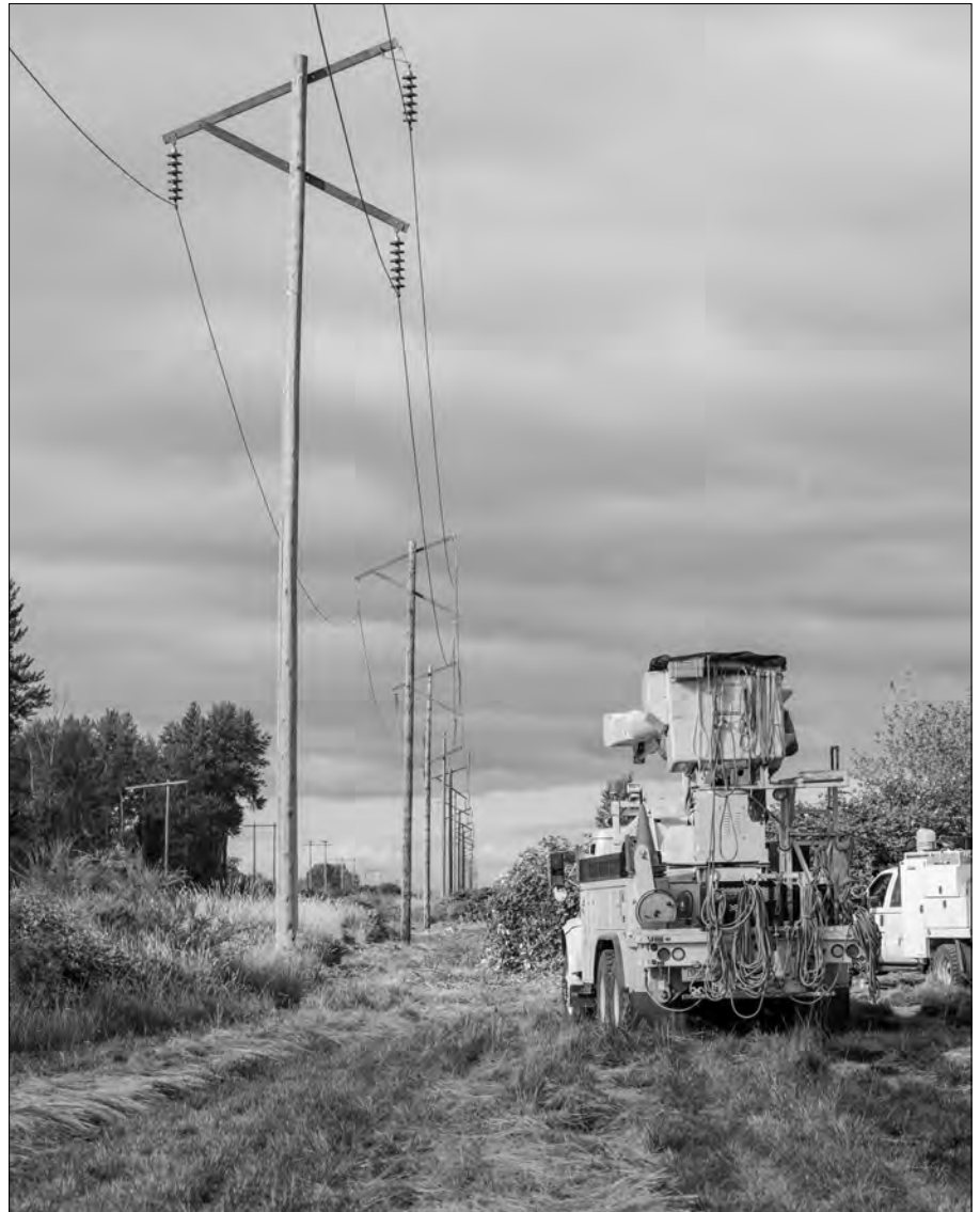
Bonneville Power Administration crews clear the right-of-way along a transmission corridor. Keeping the corridor free of trees and vegetation reduces the risk of outages and reduces fire danger.
