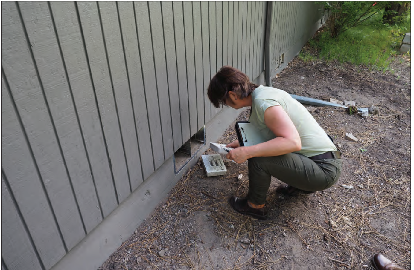
CEC Energy Specialist Jody Howe removes the plugs from foundation vents.
