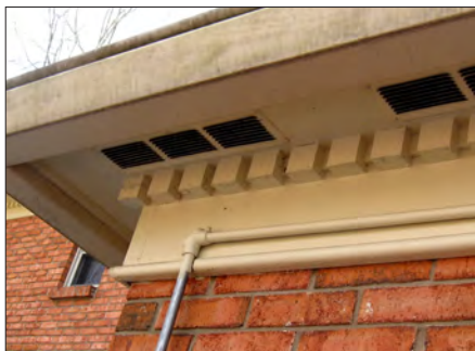
Install half of the required vent area in soffit vents. These are 4-by-16-inch vents.
