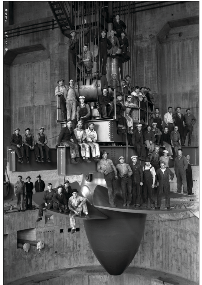
Workers on giant turbine being lowered into Bonneville Dam in 1937.
