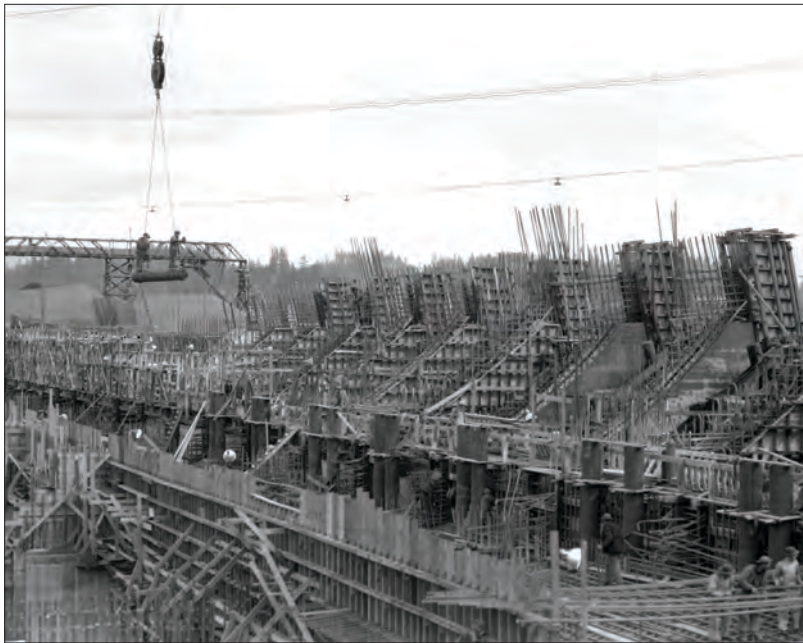
Bonneville Dam under construction in 1935.
