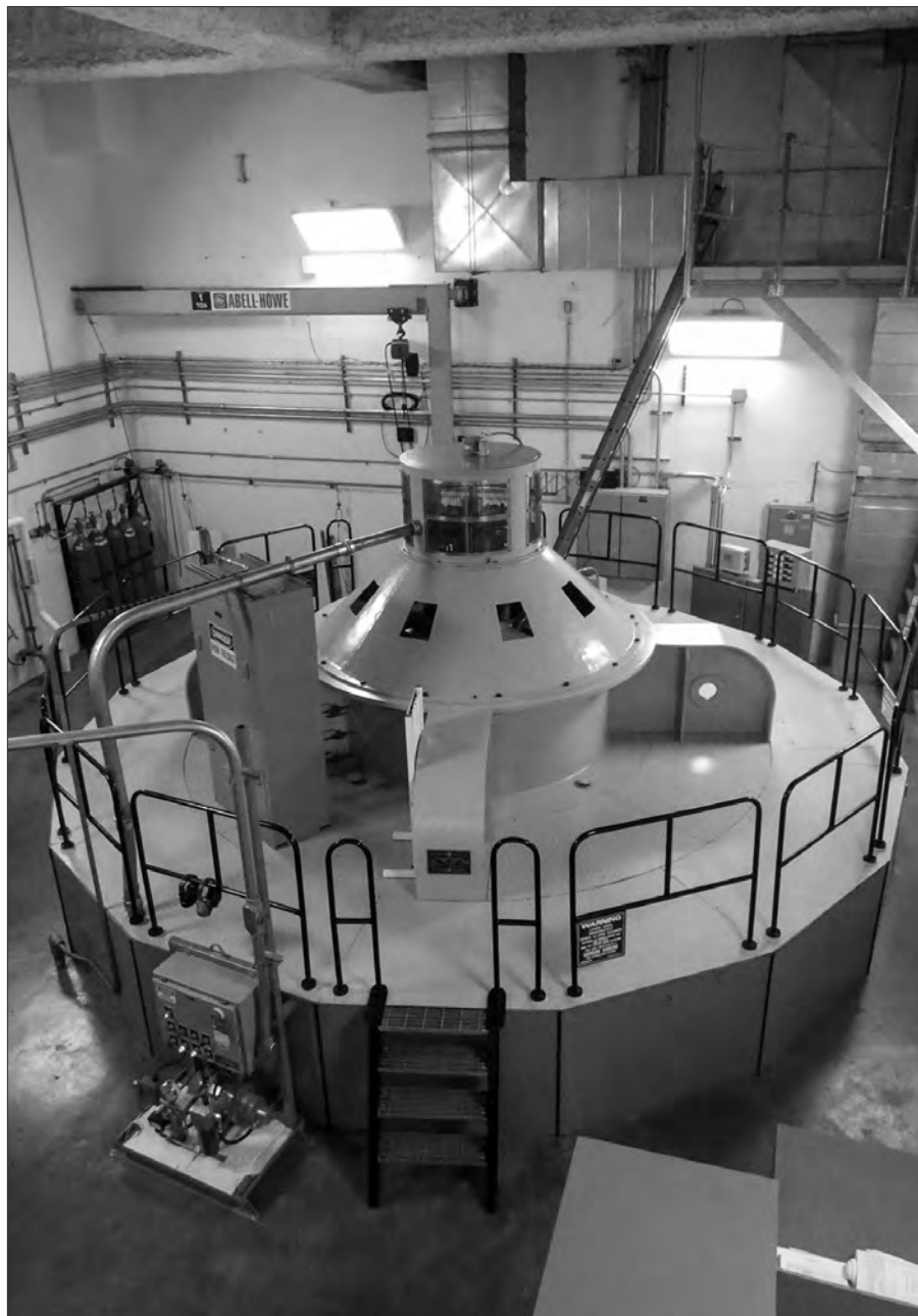
A distant view of the turbine housing at McNary Dam.
