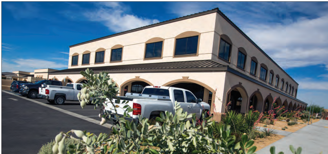
VEA's dispatch and engineering center in Pahrump earned LEED Gold Certification, which is unusual in a rural area, according to the U.S. Green Council.
