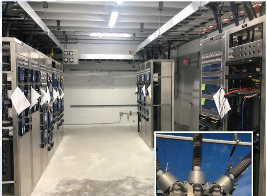
Upgrading the protection and controls at the Marathon substation included turning an old office building into a state of the art relay room. The equipment in this room enables the power load to be instantly redirected to other devices should a fault occur.
