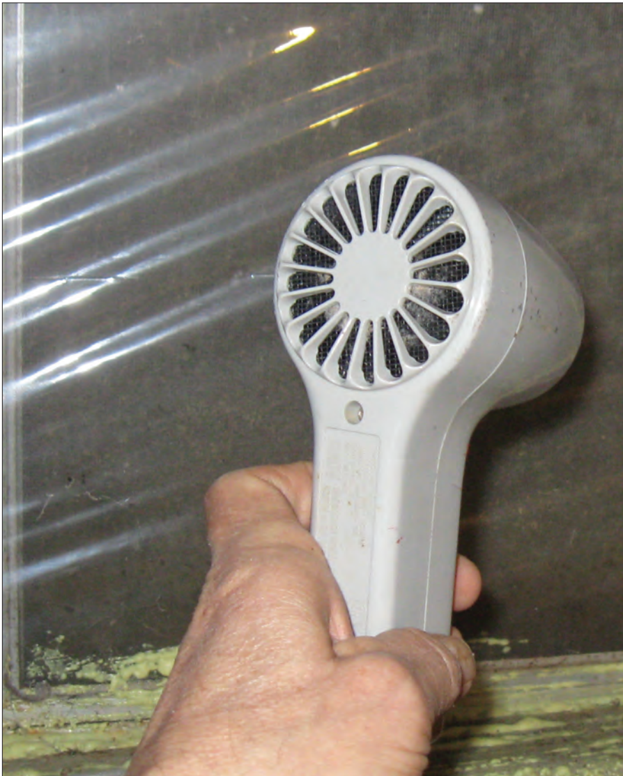
Installing clear plastic on windows during winter months is easy, and can reduce heat loss and air leaks.
