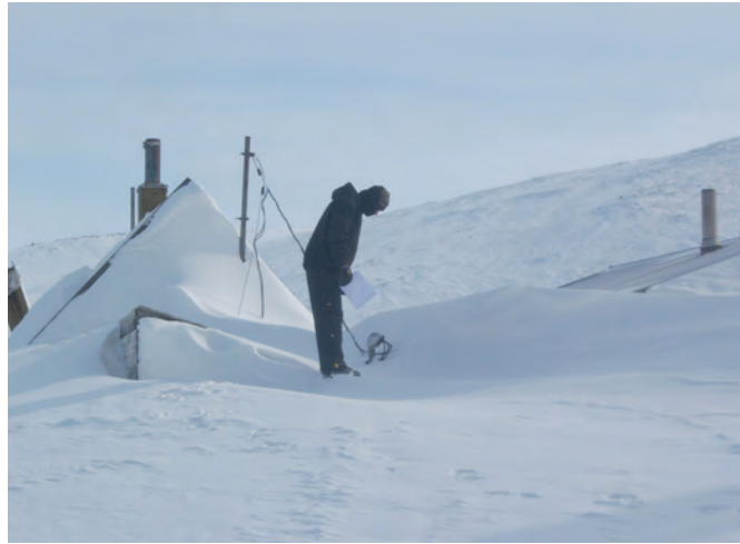
ABOVE: AVEC linemen sometimes have difficulty locating service entrances when roofs are covered with wind-blown snow.
