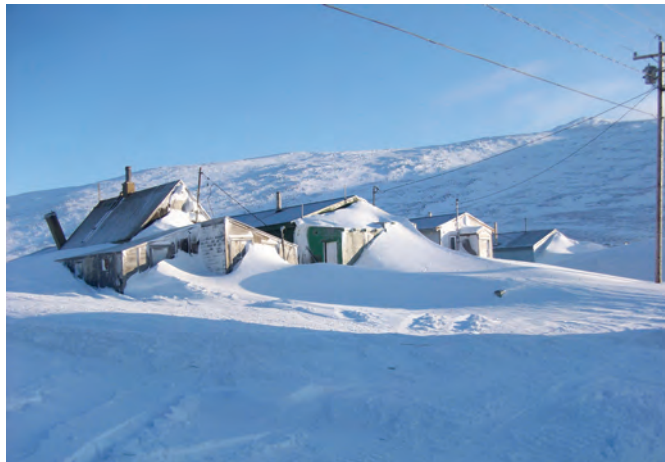
Strong winds and heavy snow storms can cause snow drifts to build up and almost cover homes, meters and service entrances.
