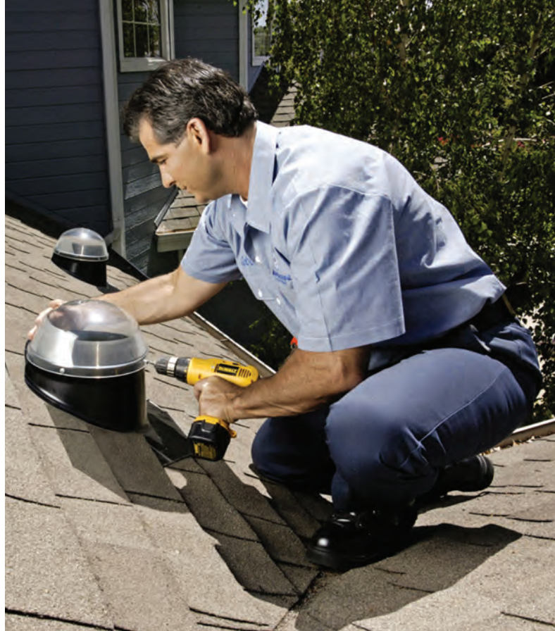
A tubular skylight is installed on a shingle roof. Notice how the shingles fit over the flashing to eliminate leaks.
