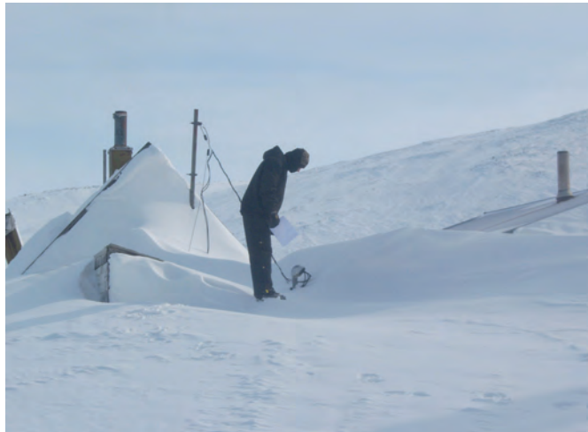
ABOVE: AVEC linemen sometimes have difficulty locating service entrances when roofs are covered with wind-blown snow.
