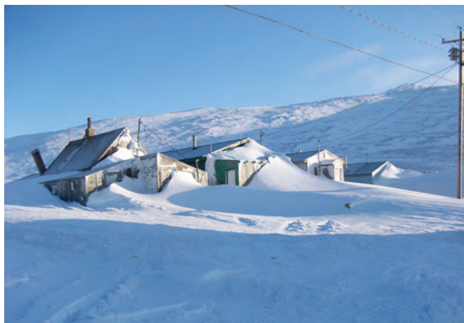
Strong winds and heavy snow storms can cause snow drifts to build up and almost cover homes, meters and service entrances.
