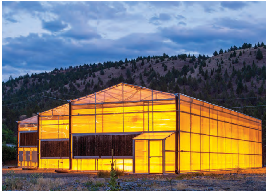
The city of John Day built a hydroponic greenhouse that uses reclaimed wastewater to grow vegetables for local stores and restaurants. PHOTO COURTESY CITY OF JOHN DAY
