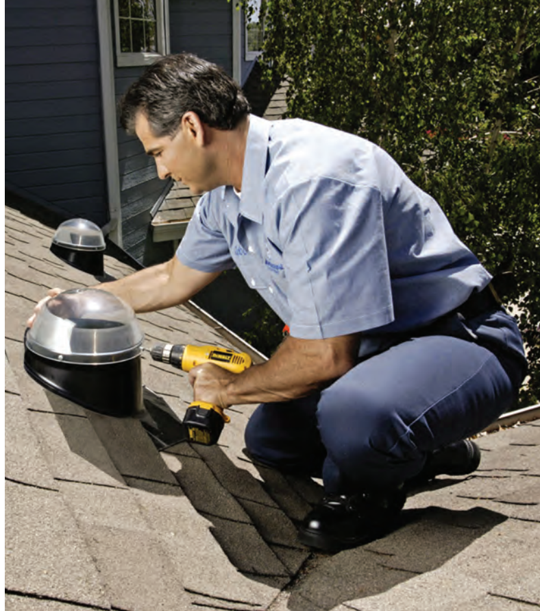
A tubular skylight is installed on a shingle roof. Notice how the shingles fit over the flashing to eliminate leaks.
