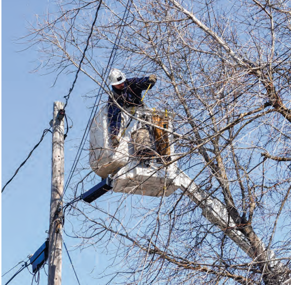
Travis clears tree branches encroaching on a power line.
