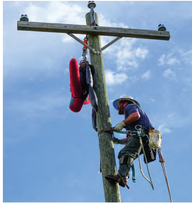
Kyle Strickling practices pole-top rescue during a safety training session for line crews.
