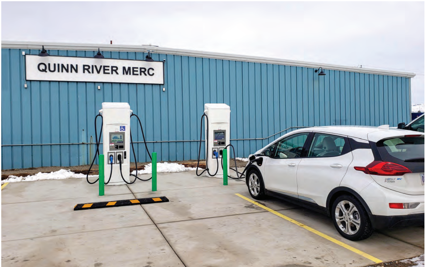
The McDermitt electric vehicle charging station is at the Quinn River Merc. It can take from 30 minutes to an hour to charge an EV at these newly installed fast chargers. PHOTOS COURTESY OF HARNEY ELECTRIC COOPERATIVE
