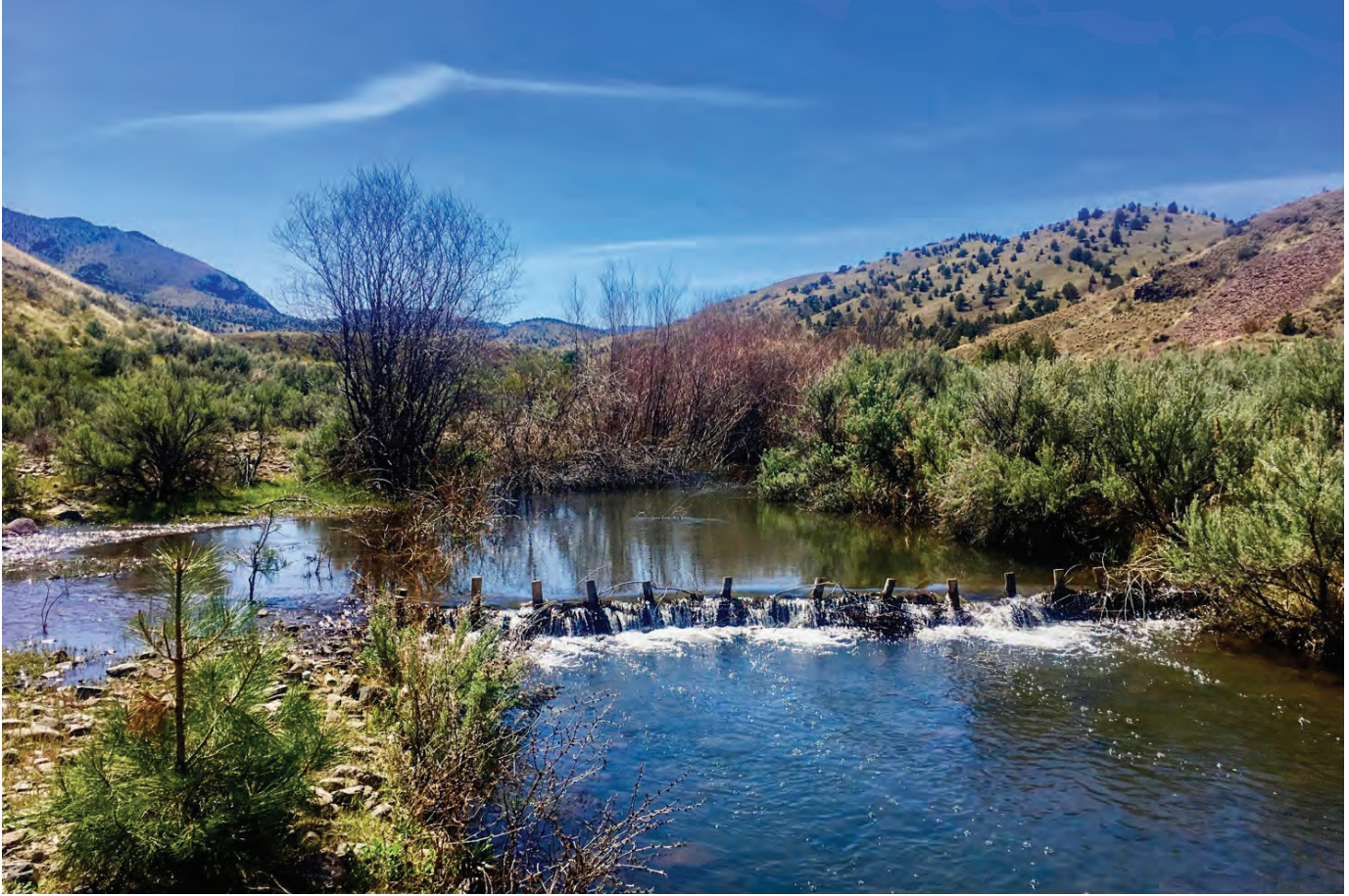
Beaver dam analogs are channel-spanning, permeable structures built with woody debris and fill material to form a pond and mimic natural beaver dams. PHOTO COURTESY OF HERB WINTERS
