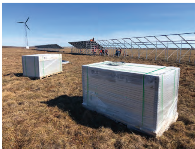
ABOVE AND OPPOSITE PAGE: An Alaska Native Renewable Industries crew installs photovoltaic modules on racking.
