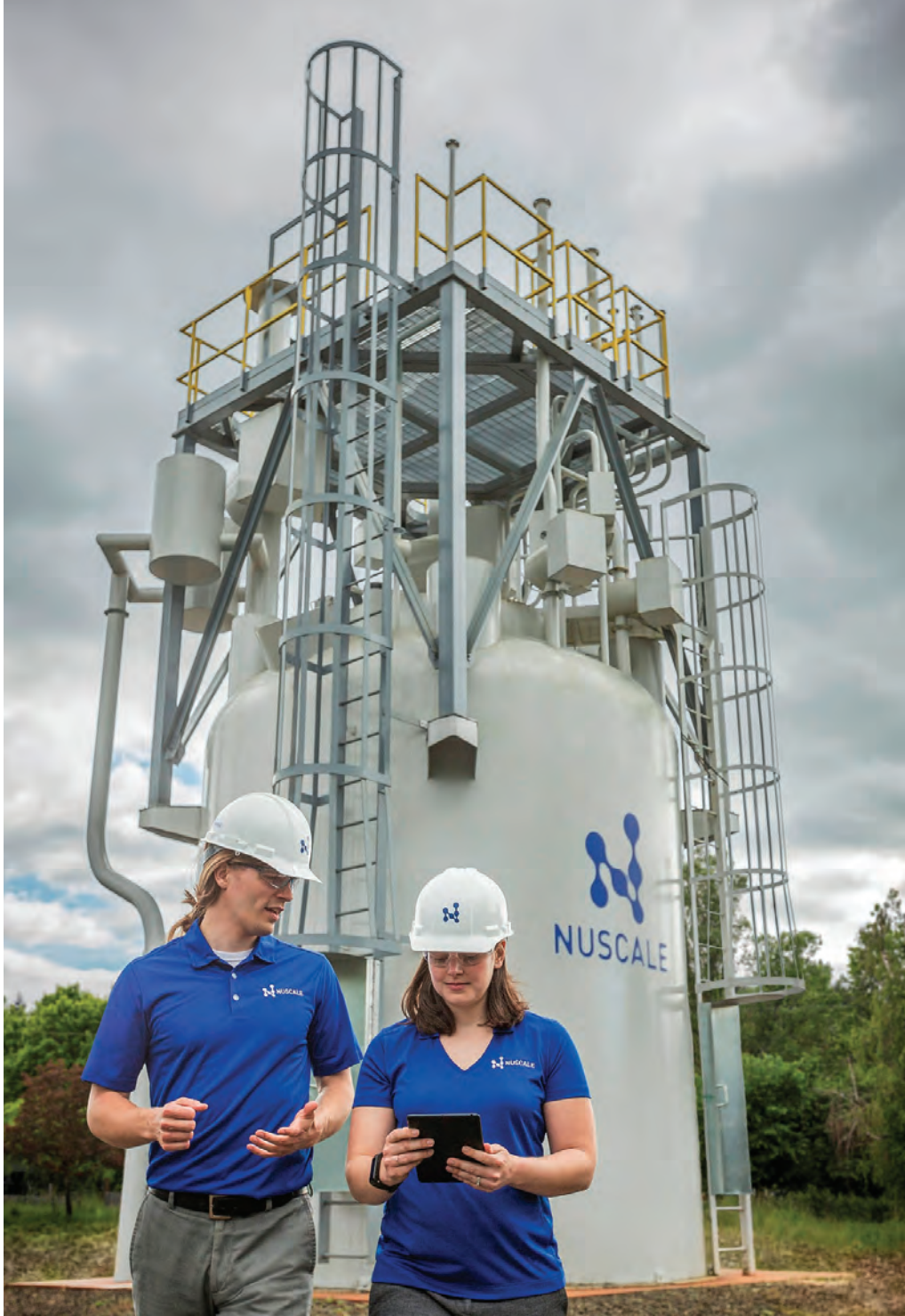
The upper third of a NuScale Power module prototype in Corvallis, Oregon. Two-thirds is underground. A traditional nuclear reactor can be 208 feet high and 131 feet wide. A small reactor is closer to 76 feet high and 15 feet wide. PHOTOS COURTESY OF NUSCALE POWER
