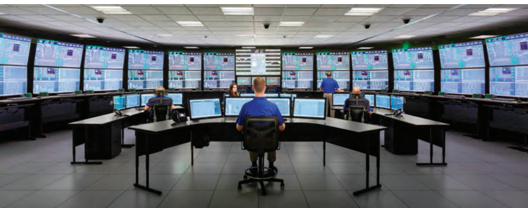
NuScale’s control room simulator prepares operators to monitor the small modular reactors.
