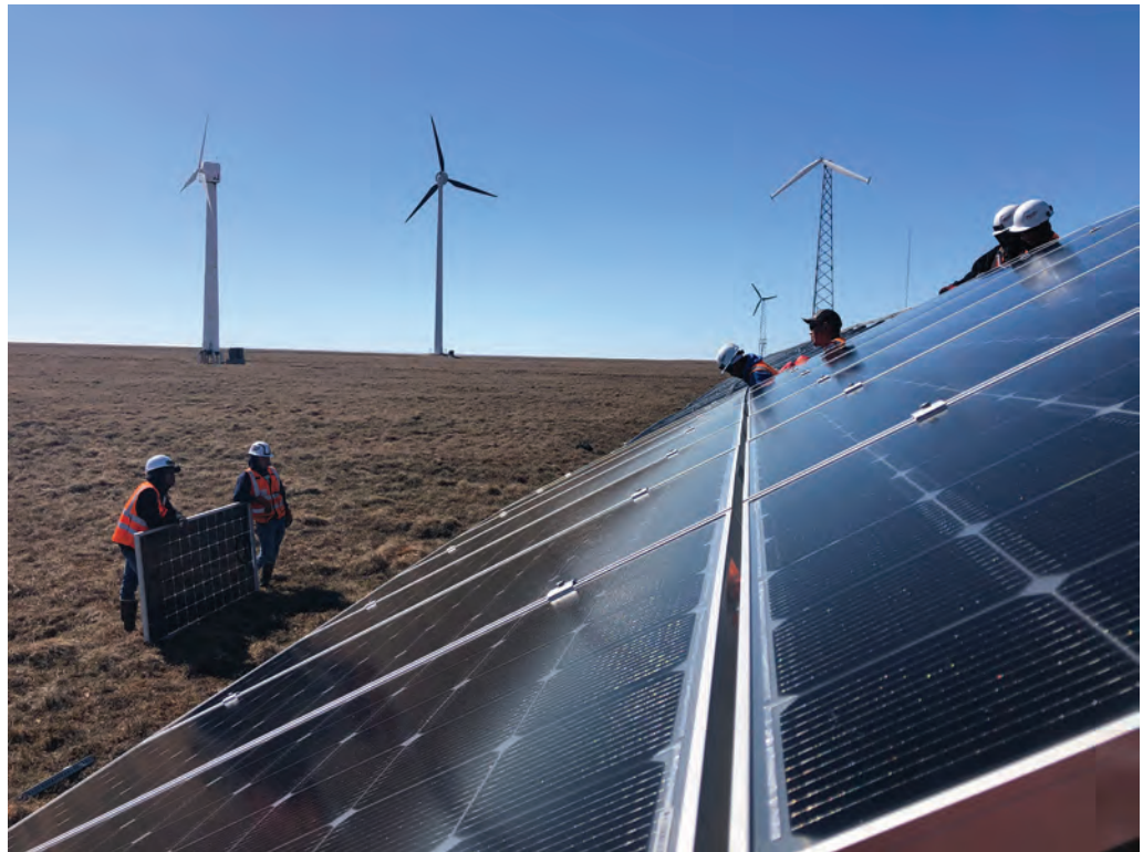
ABOVE AND OPPOSITE PAGE: An Alaska Native Renewable Industries crew installs photovoltaic modules on racking.
