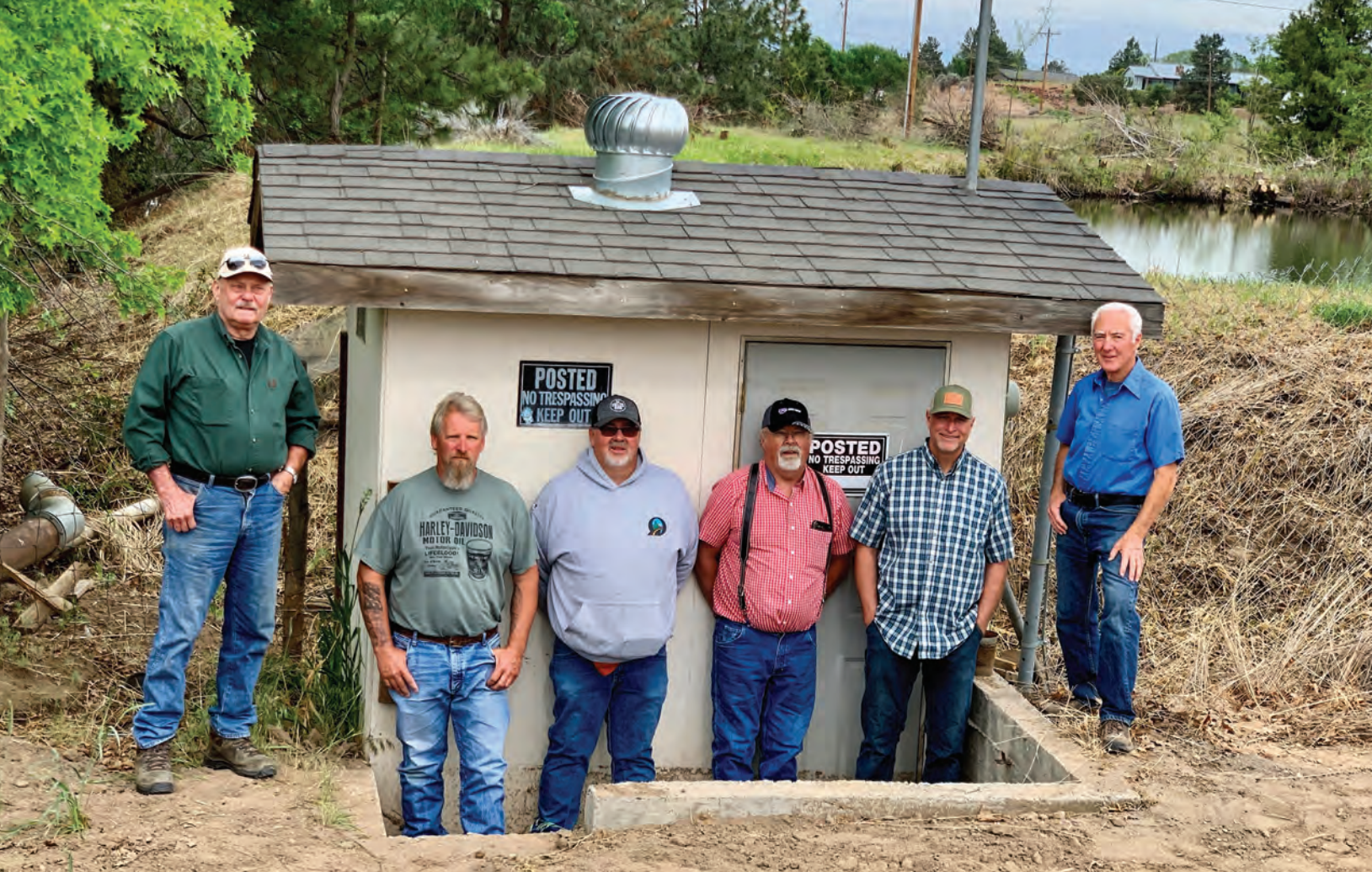
The board members who brought forth the variable frequency drive project stand outside the Bierly Acres pump house. From left are former board member Ron Lindquist, Mark Jensen, Floyd Paye, Duane Fuller, Dan Comingore and Chuck Alexander. PHOTOS COURTESY OF DAN COMINGORE
