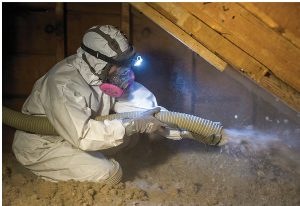
ABOVE: Loose-fill insulation is a good approach for insulating your attic floor. BELOW: It's a good idea to seal air leaks before you add more insulation. PHOTOS COURTESY OF THE DEPARTMENT OF ENERGY
