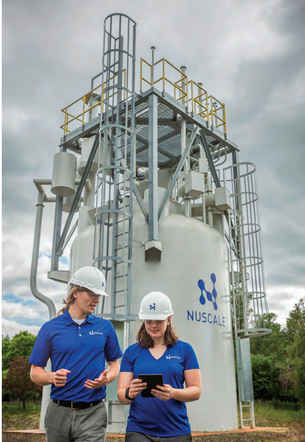
The upper third of a NuScale Power module prototype in Corvallis, Oregon. Two-thirds is underground. A traditional nuclear reactor can be 208 feet high and 131 feet wide. A small reactor is closer to 76 feet high and 15 feet wide. PHOTOS COURTESY OF NUSCALE POWER
