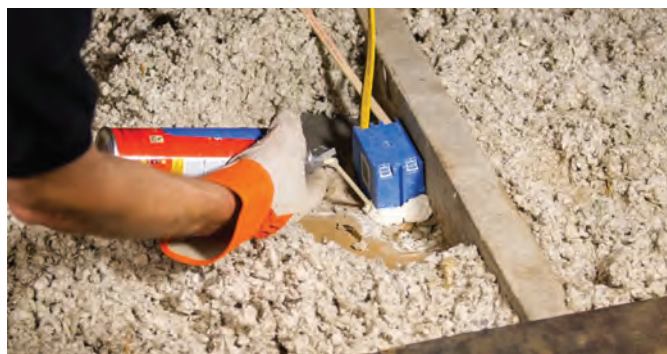
ABOVE: Loose-fill insulation is a good approach for insulating your attic floor. BELOW: It's a good idea to seal air leaks before you add more insulation. PHOTOS COURTESY OF THE DEPARTMENT OF ENERGY
