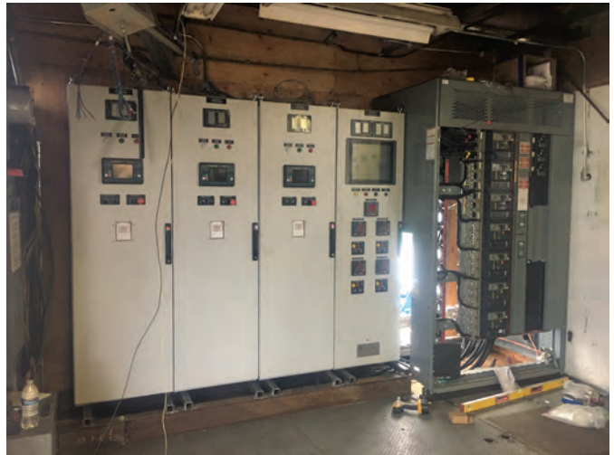
ABOVE: A new automated switch gear, control panels and master panel will soon power Shungnak and Kobuk.
