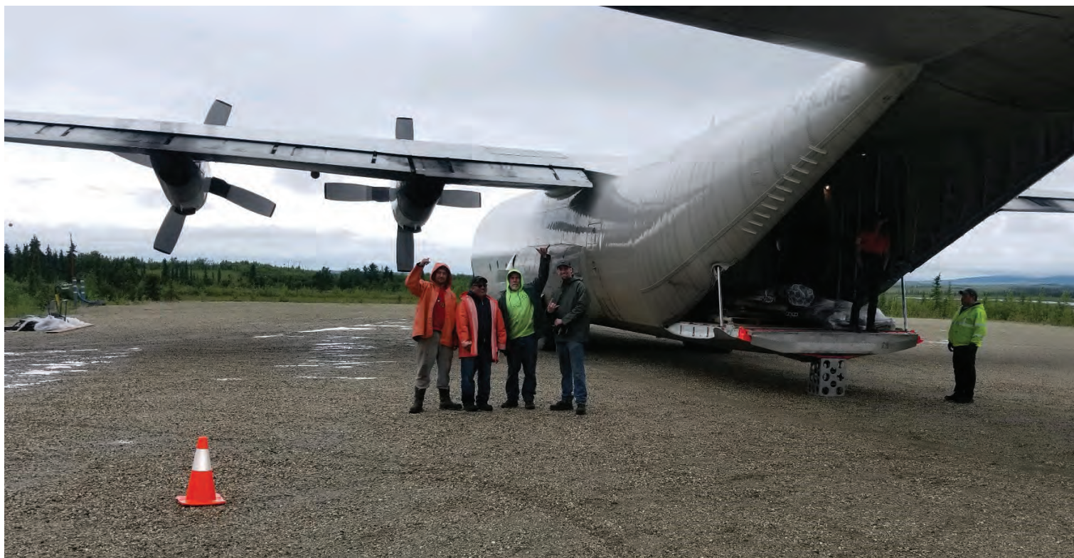
Alaska Village Electric Cooperative crew members unloaded 30,000 pounds of freight for the Shungnak power plant project to upgrade to automated switchgear. From left, Don deLima-Schou, Ciro Rivera, Bob Washington and Patrick Shick. The aircraft is a C-130 Hercules flown by Lynden Air Cargo. PHOTO COURTESY OF PATRICK SHICK
