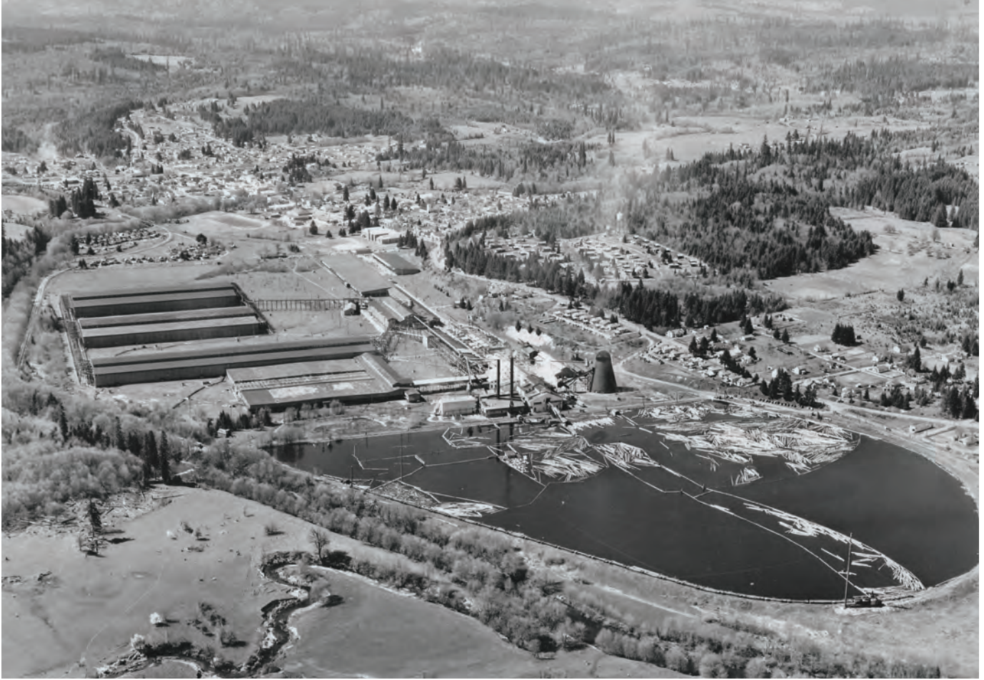
The Oregon-American mill site in Vernonia covered more than 200 acres. The 36-acre mill pond is in the foreground of the photo. The town of Vernonia is above the mill site. PHOTO COURTESY OF THE VERNONIA PIONEER MUSEUM
