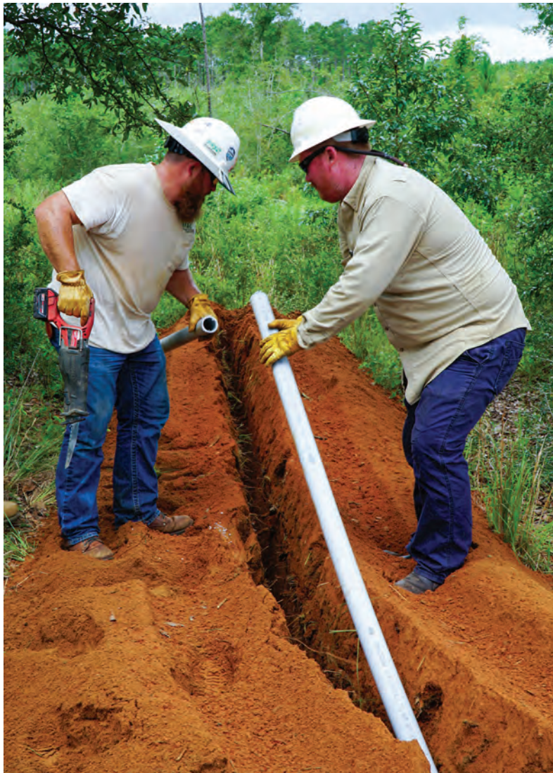
ABOVE: Wesley Clark, left, and Tony Moody fit underground pipe that will house electric lines. BELOW: Underground electric lines eventually have to come up for air. Tony connects an underground service to the overhead power system.
