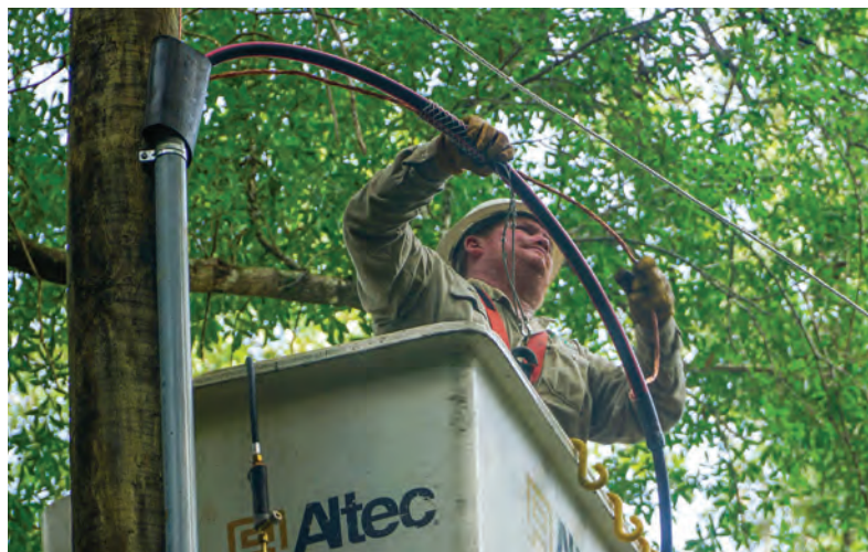
ABOVE: Wesley Clark, left, and Tony Moody fit underground pipe that will house electric lines. BELOW: Underground electric lines eventually have to come up for air. Tony connects an underground service to the overhead power system.
