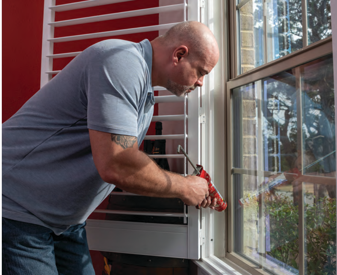
Use caulk to seal gaps around non-moving parts of doors and windows. PHOTO BY SCOTT VAN OSDOL
