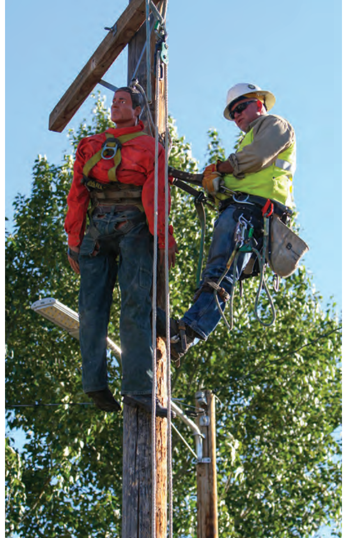
Oregon Trail Electric Cooperative Lineman Jeremy Adair participates in pole-top rescue training in John Day. PHOTO COURTESY OF OTEC
