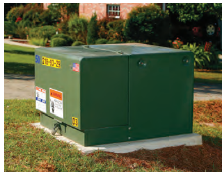
ABOVE: Pad-mounted transformers route large amounts of electricity. Only utility lineworkers and crews should be near them. RIGHT: If you decide to plant landscaping around transformers, respect the required safe clearance zone at plant maturity.
