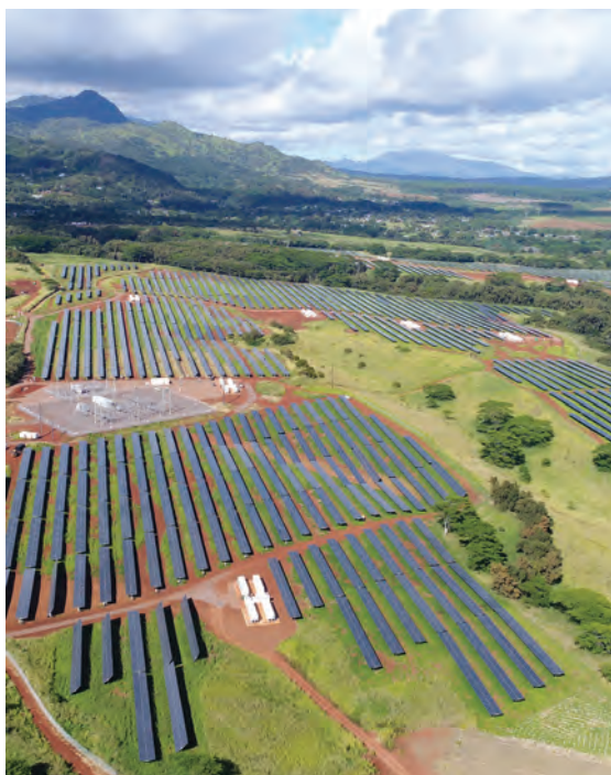
AES Distributed Energy worked with Kaua'i Island Utility Cooperative on the world's largest operational solar-plus-storage system. The 28-megawatt solar plant in Lawai is connected to a 100-megawatt-hour battery energy storage system, providing cheap, clean energy when it is most valuable, instead of just when the sun shines. PHOTO COURTESY OF AES
