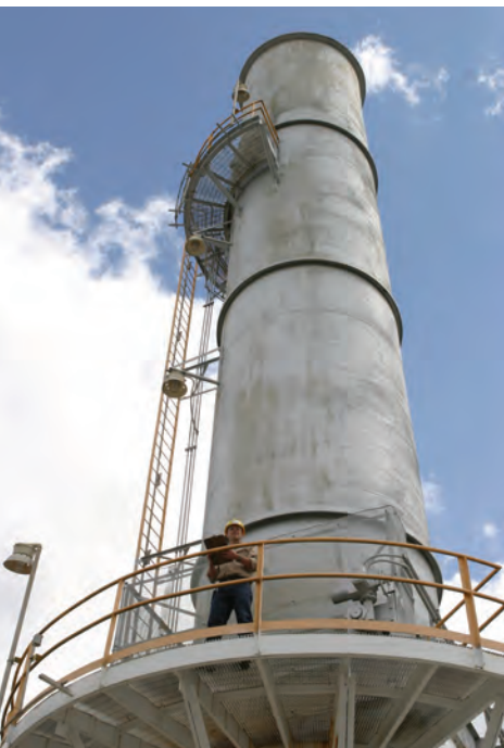
The McIntosh natural gas-fired plant is a cornerstone of PowerSouth's energy supply. PHOTO BY POWERSOUTH ENERGY COOPERATIVE
