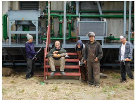
Mekoryuk crews renovate the power plant by removing rust and adding new paint.
