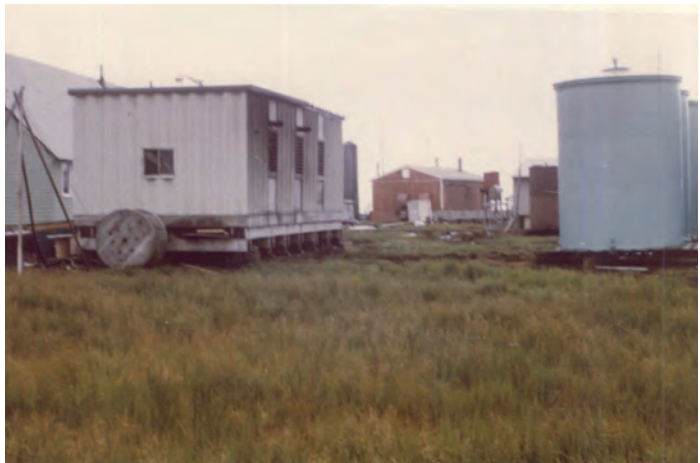
Savoonga's original power plant and bulk fuel tank farm.
