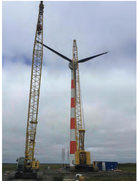
A new wind turbine goes up in Bethel.
