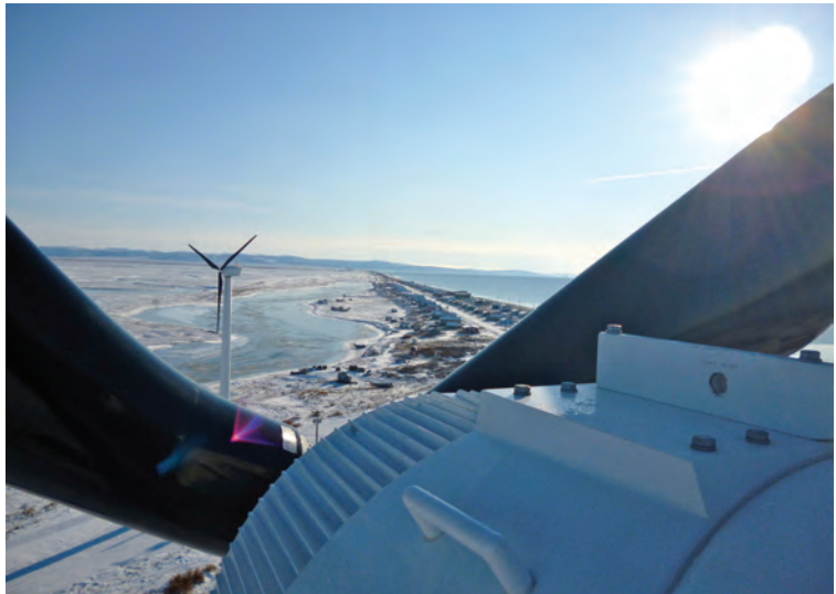
An aerial view from the top of a Shaktoolik wind turbine.
