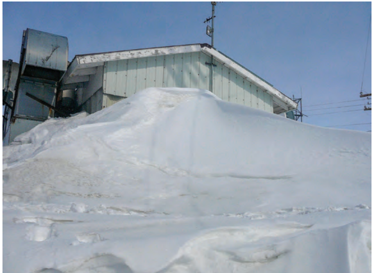
Deep snow covers the Wales power plant.
