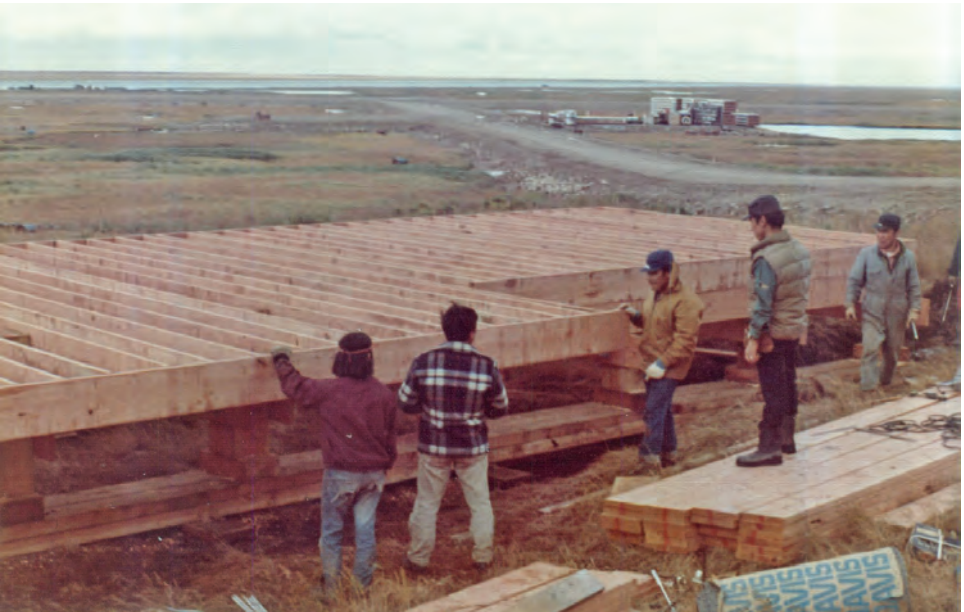
Building the foundation for Scammon Bay's power plant.
