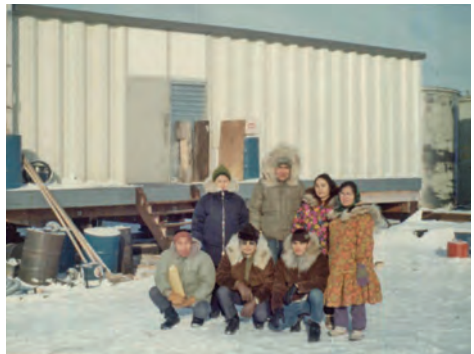
The Stebbins power plant in the early years.
