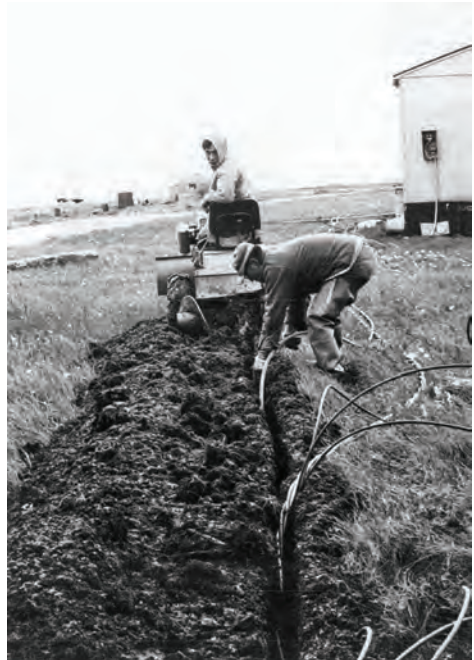
Richard Nanuk and Clarence Smith install underground wiring.
