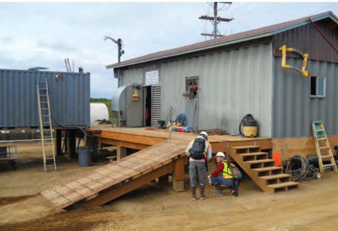
New Stuyahok power plant renovation.
