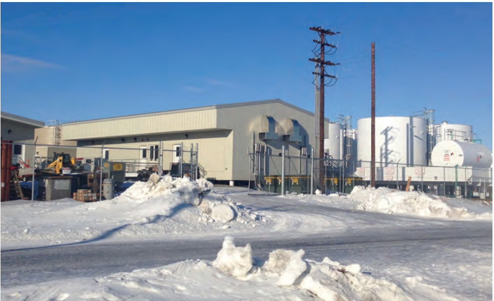
The Stebbins power plant and bulk fuel tank farm.
