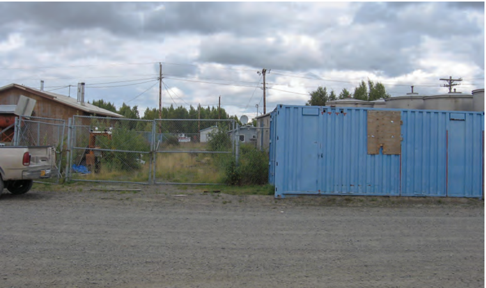
The retired Lower Kalskag power plant.
