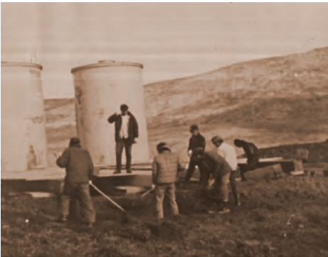
Manual labor and old-school methods were used to build the original power plants.
