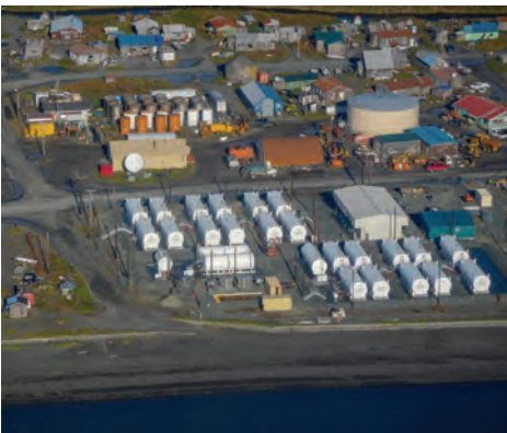
Togiak's power plant and bulk fuel tank farm.
