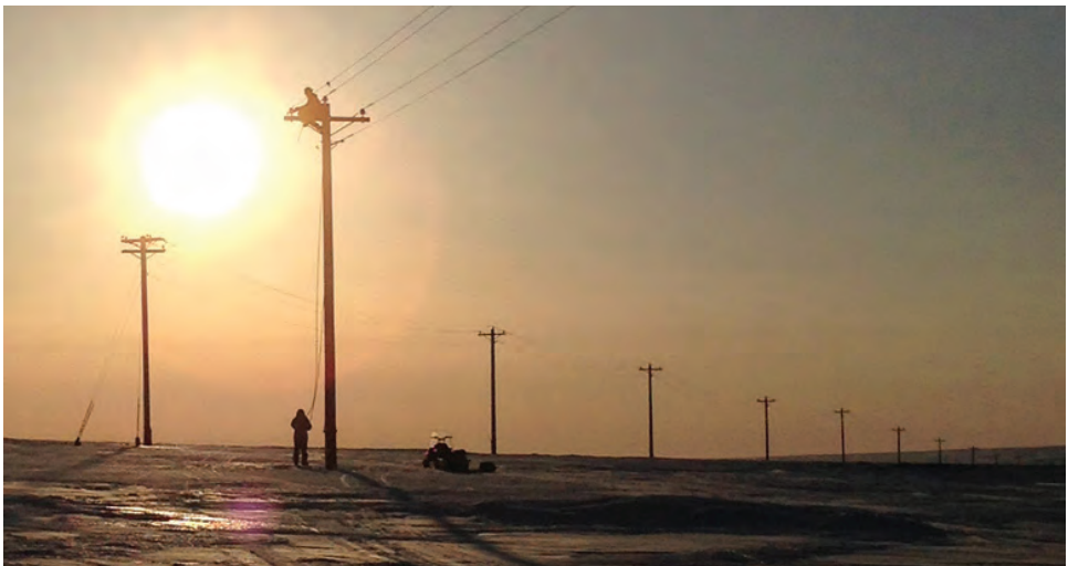
A crew works on the intertie between Toksook Bay and Tununak.
