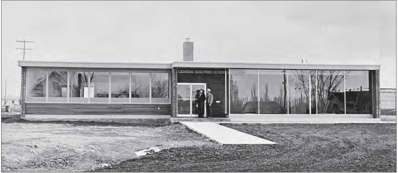
In 1950, Central Electric Cooperative relocated into a new headquarters on Highland Avenue in Redmond for $48,000.
