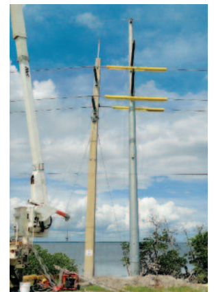
Hurricane Donna destroyed over 100 utility poles in 1960. Since then poles have improved and FKEC now implements ductile iron poles rated to withstand 150 m.p.h. winds.
