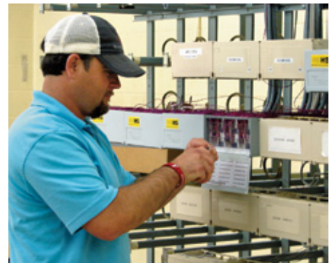
RYAN HIGDON changing cable pairs in Flat Rock.
